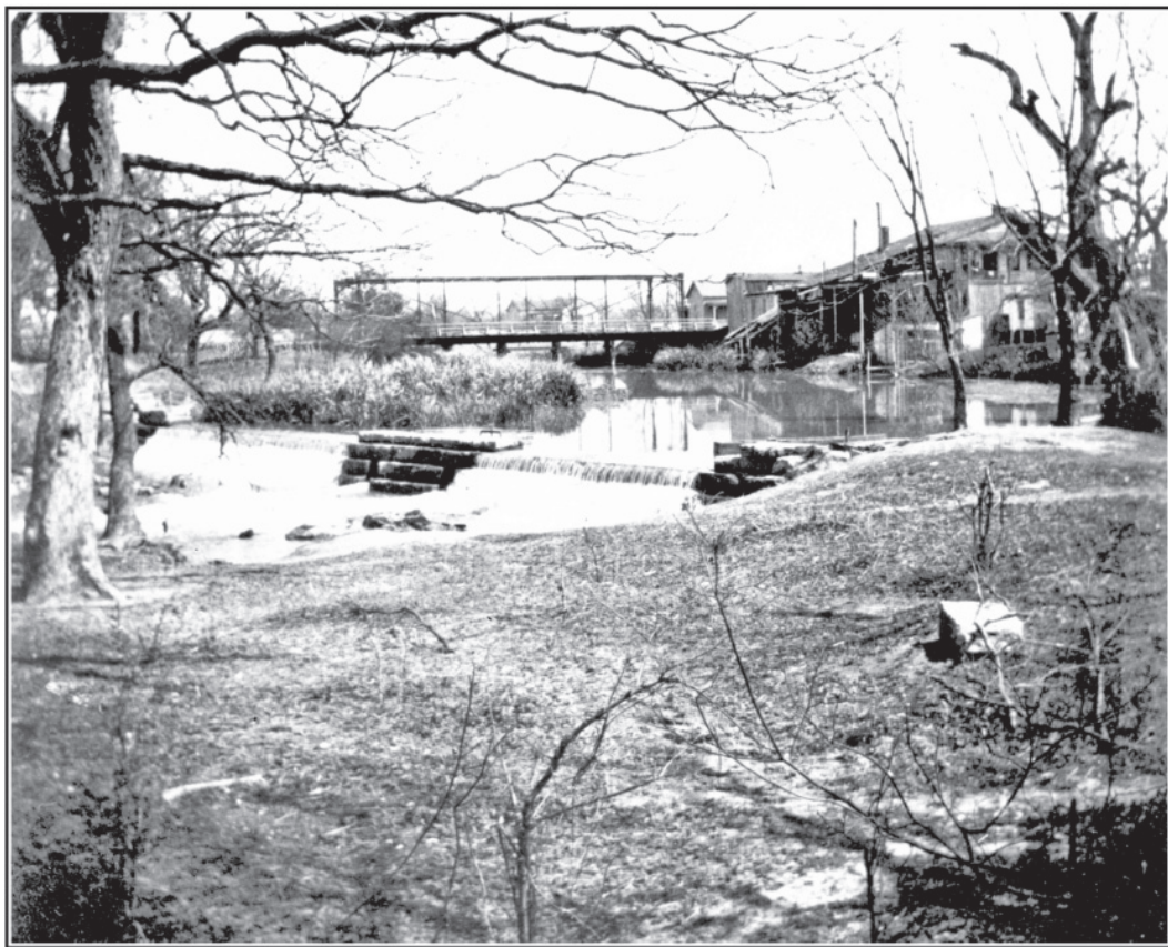
Figure 4-7. Circa 1893 photograph of the Alamo Mills Dam. Note Grand Avenue (later Jones Street) Bridge in the background. Facing NE.
