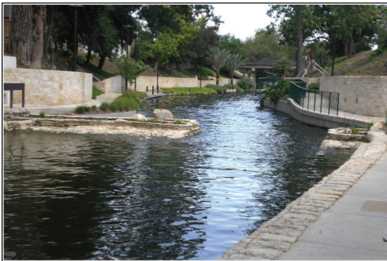
Figure 6-2. The Lexington Avenue Dam after the portion was removed to allow for river barges to pass to the newly improved section of the Riverwalk.
