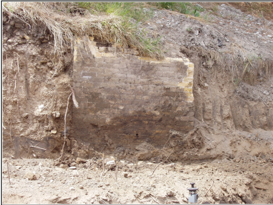
Figure 4-17. Feature 6, yellow brick wall (see Figures 4-1 and 4-12).
