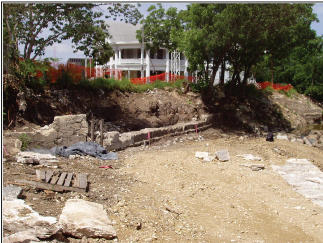
Figure 4-10. View of Alamo Mills Dam and adjoining retaining wall.
