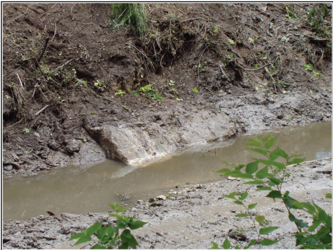
Figure 4-3. Alamo Mills Dam (41BX1817) when first encountered.
